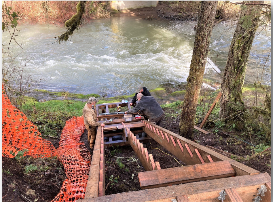
Linn County Parks employees work on the steps down to Thomas Creek at the new Bilyeu Den Park next to the Hannah Covered Bridge near Scio.
