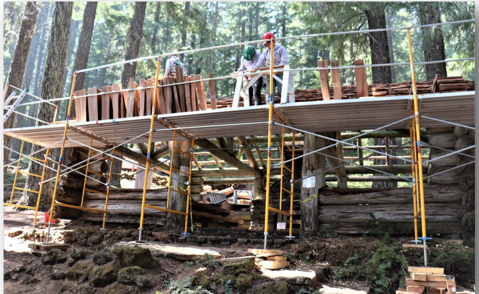
HistoriCorps volunteers install hand-split cedar shakes on the picnic shelter at Clear Lake Resort.
