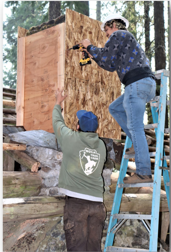
Above: Jason Benson and Remy Buxton, on ladder, work on the fireplace at the Clear Lake picnic shelter.
